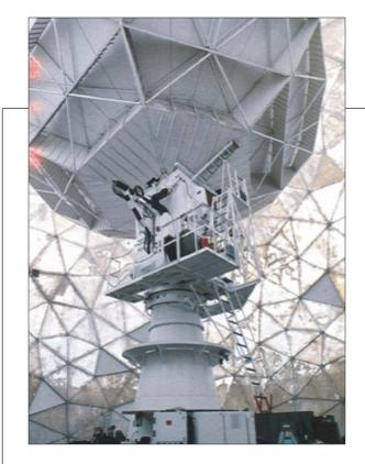
The ARPA-Lincoln C-band Observables Radar (ALCOR) became operational. ALCOR was the first high-power microwave radar to utilize wideband waveform transmissions. ALCOR's goals were to develop the technology necessary to generate and process wide-bandwidth signals and to investigate the applications of broadband data for reentry vehicle discrimination and space situational awareness.
