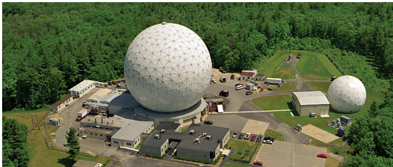
FIGURE 1. The Haystack antenna is the largest radome-enclosed antenna in the world. The radome protects the fragile antenna from wind and snow loading, and prevents distortion of the antenna surface caused by wind, snow, and sun. The radome does cause slight attenuation of the radio waves passing through it, but the stability and reliability that the radome ensures more than compensates for this slight downside.
