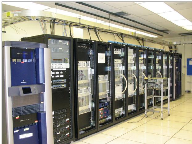
**FIGURE 16.** Reduced complexity and reduced costs were realized by having a common set of eleven racks for each radar.
