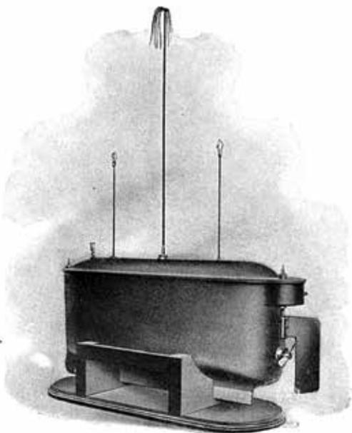
**FIGURE 1.** In addition to a radio antenna (center), Tesla's iron-hulled radio-controlled model boat included a pair of elevated lights to assist an on-shore operator with keeping the vessel on course at night [2].
