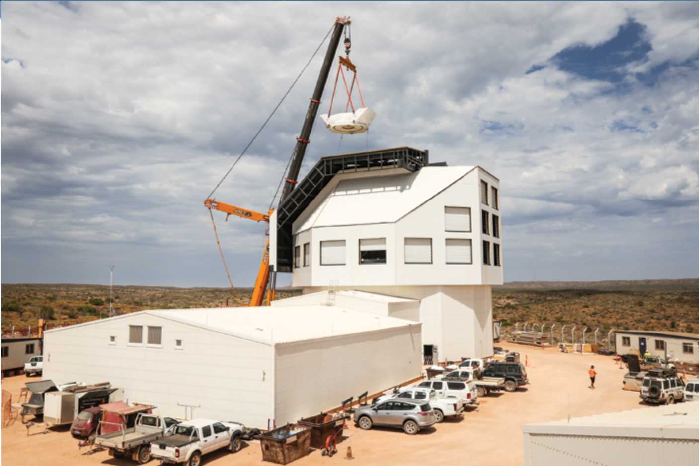
The Space Surveillance Telescope mount installation is underway in the newly completed enclosure in northwest Australia.
