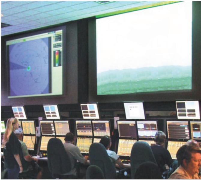
FIGURE 5. The modernized mission command-and-control center at RTS remains in use.
