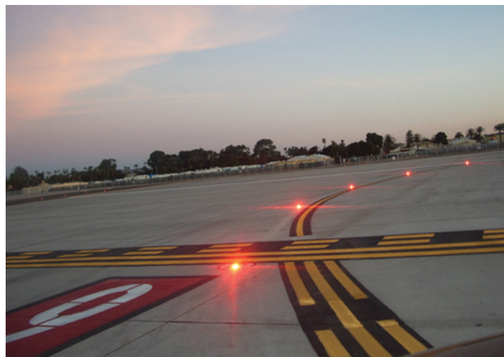
Figure 1. The RWSL warning signals illuminate red when a runway or intersection is unsafe for an aircraft to enter.
