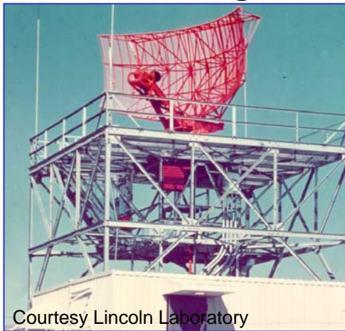
Airport Surveillance Radar
