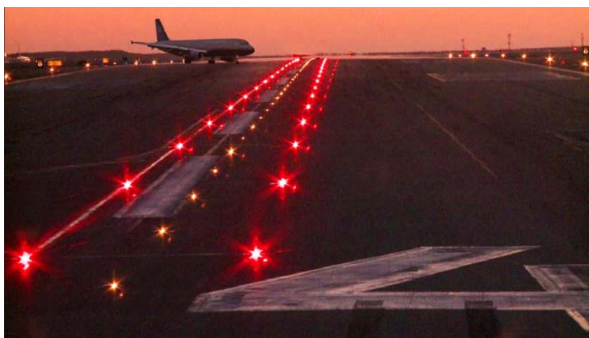
Takeoff Hold Lights indicate that there is some obstruction (in this case crossing traffic), so the pilot should hold position until the runway is cleared.
