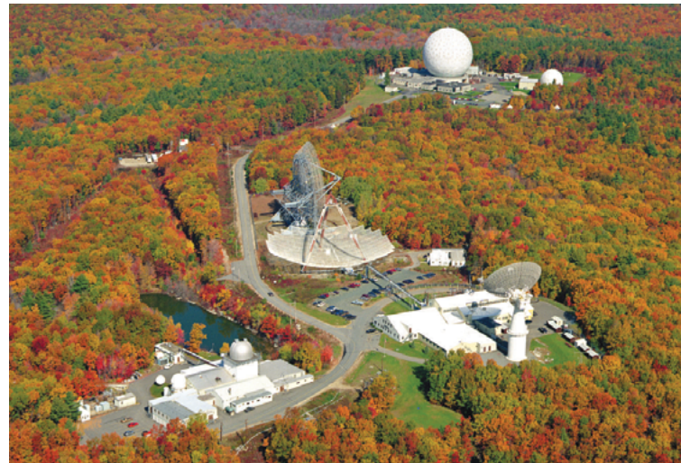
Lincoln Space Surveillance Complex, Westford, Massachusetts
