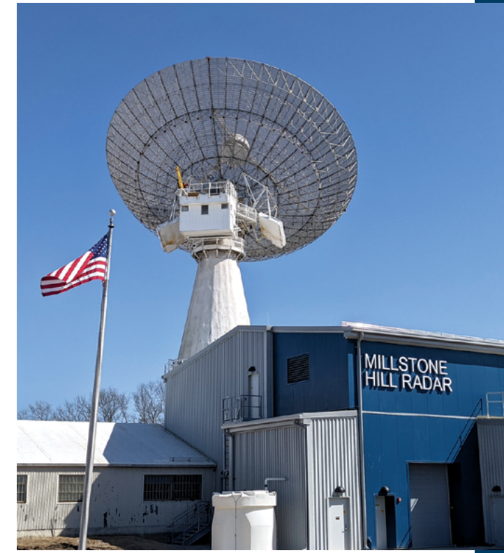
The Millstone Hill Radar, with an 84 ft antenna and 3 MW of peak power, operates at L-band (1.3 GHz) and is capable of tracking satellites in deep space 30,000 miles from the Earth and beyond.
